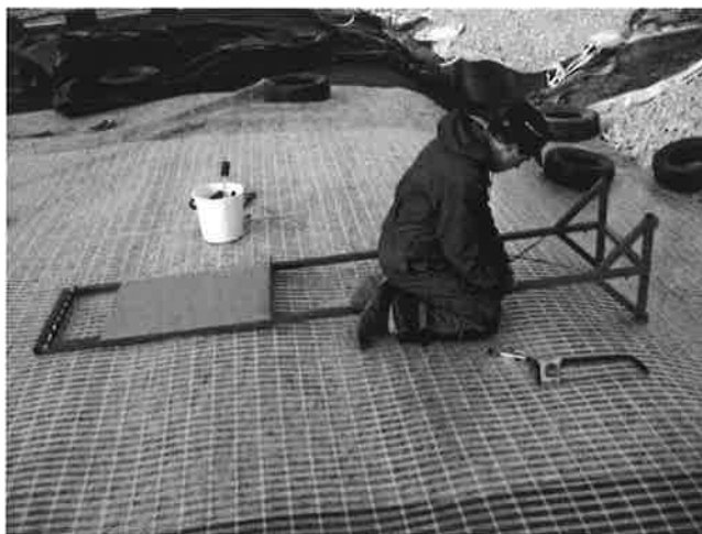
Secugrid @200/40 R6 as slope reinforcement
